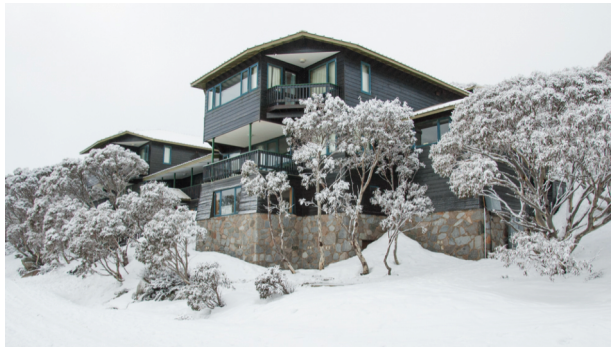
existing photo (west wing)
