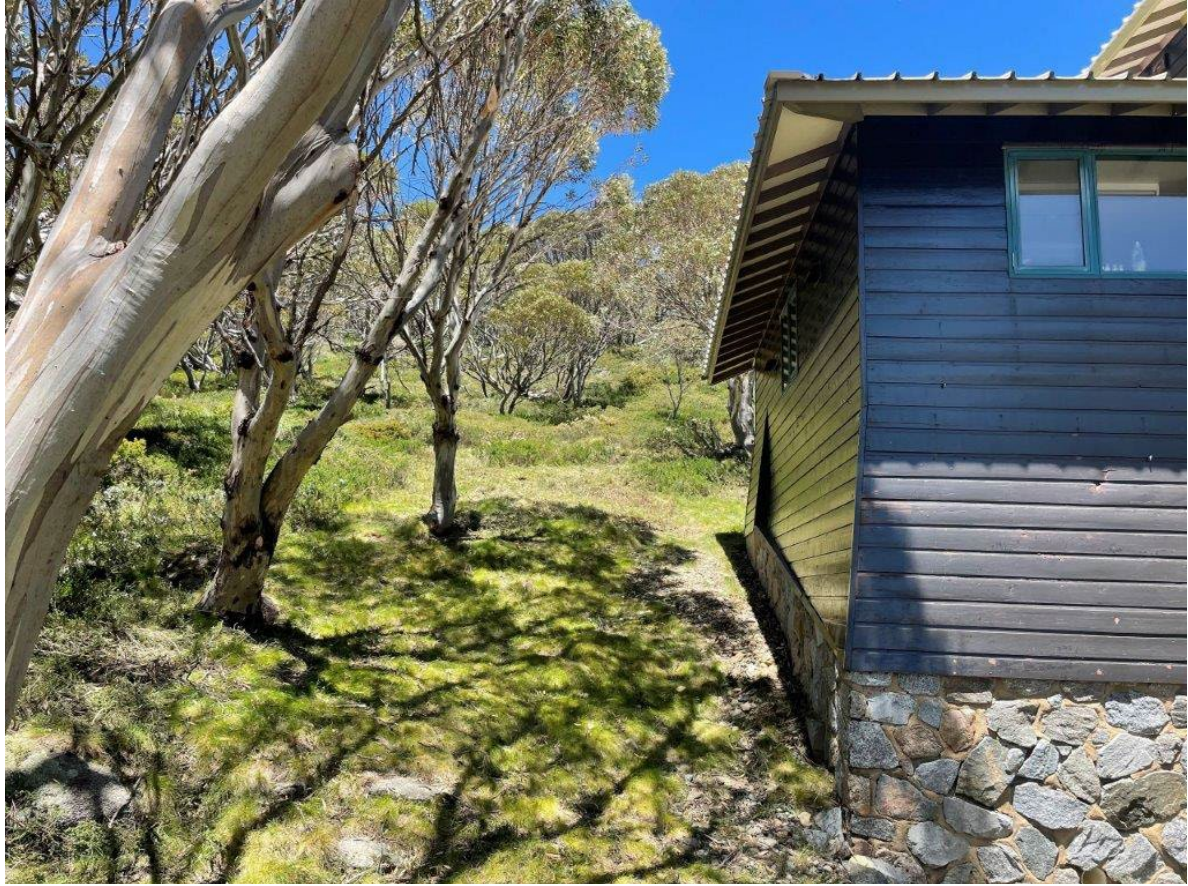
Figure 1: Typical western red cedar panels on Pygmy Possum Lodge. Photo also highlights exposed timber in eaves and timber barge boards. APZ clearance is approximately 5m to east of lodge. APZ clearance highlighted by change in ground vegetation height.
