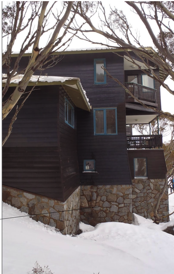
existing photo (east wing front)
