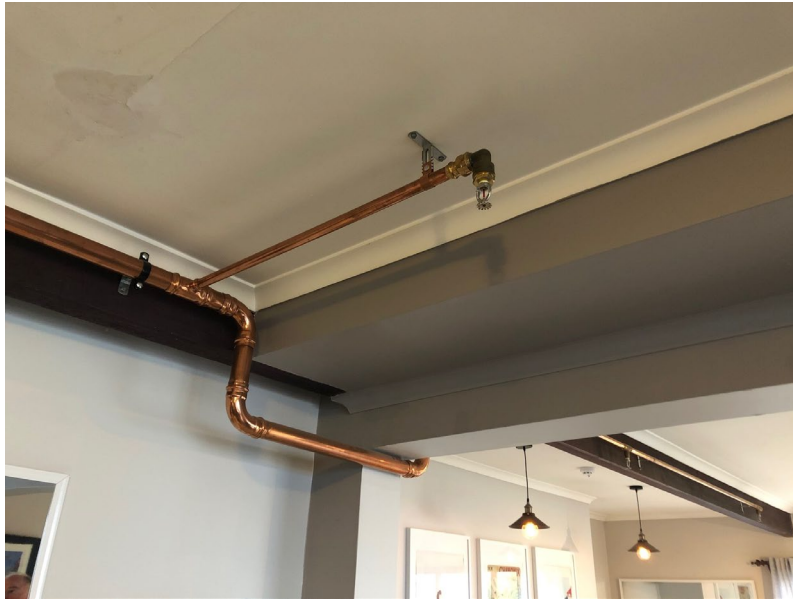
Figure 7: Installation in YCA Thredbo.
