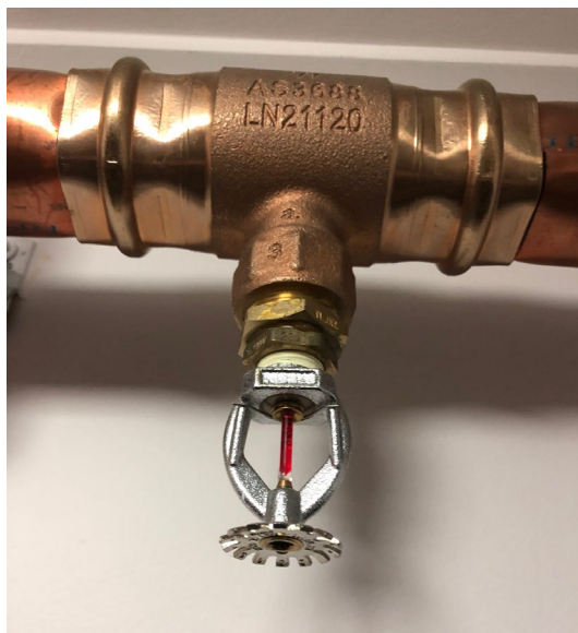
Figure 6: Example exposed copper sprinkler installation in YCA Thredbo. Glass rod breaks at 55-77°C. The glass colour indicates the temperature range. Red is a low temperature range. All joints are pressure crimps, this reduces install costs as no welding or soldering is involved
