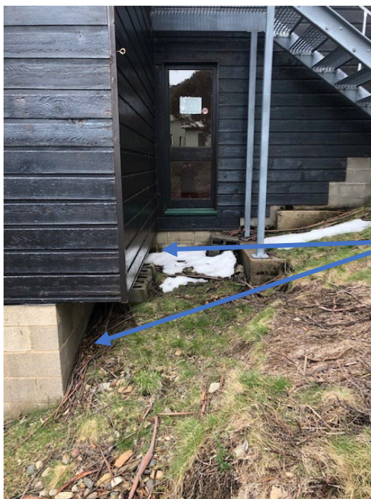
Figure 5: Minor areas requiring meshing with stainless steel 2mm aperture mesh to reduce fuel build-up. View is of the west side; a similar situation exists on the east side.
