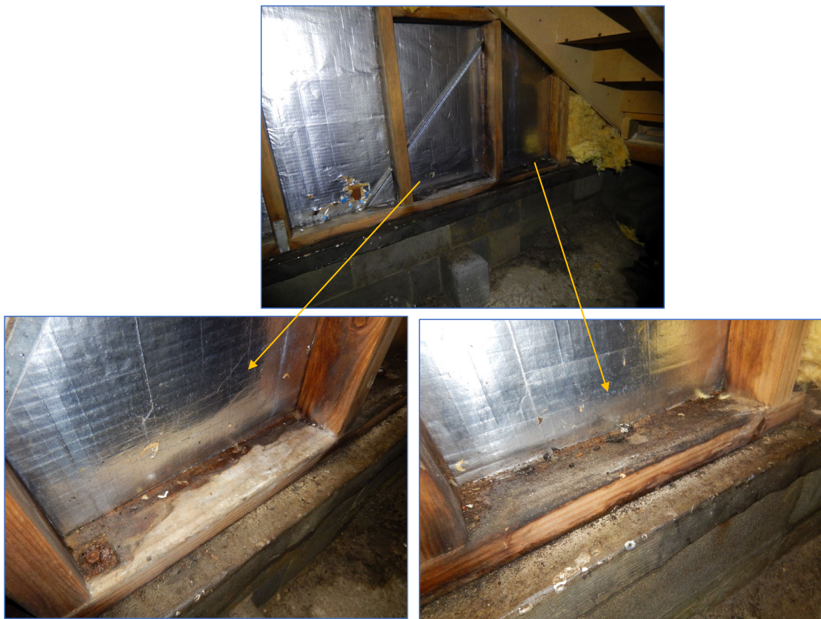
Figure3: Detail of same area highlighting moisture in frame.
