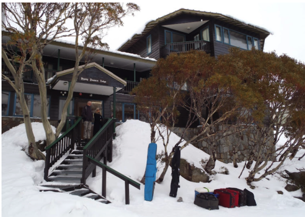
existing photo (west wing)
